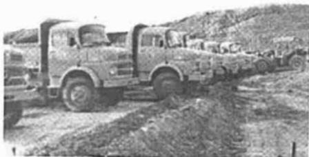
MERCEDES BENZ TIPPER TRUCKS USED FOR EARTHMOVING
